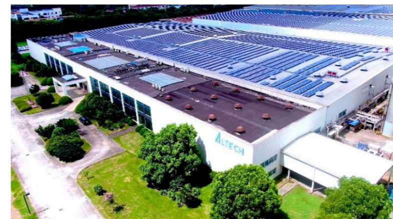
Solar panels installed at the Suzhou plant in 2021
