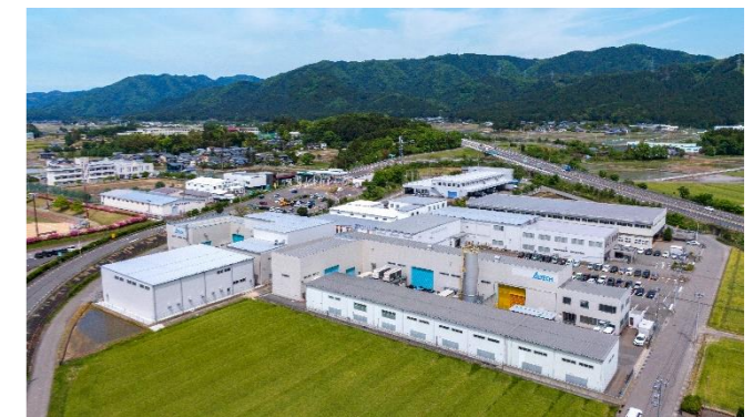
Fukui plant where solar panels will be installed
