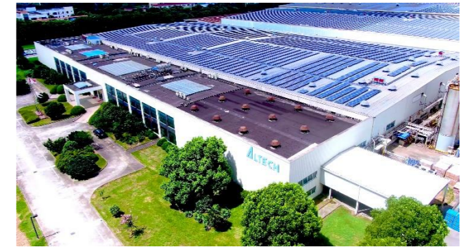
Solar panels installed at the Suzhou plant
