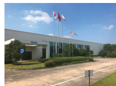
● Altech New Materials (Suzhou) Co., Ltd.
